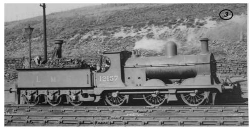
class 4F nearest the camera has been fitted with back cab protection for use on snow plough duties.
