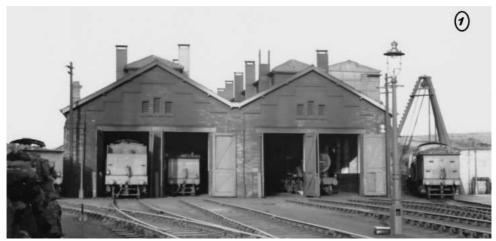
1. The ex-Midland Railway four road engine shed. To the right can be seen the water tower and also the "sheer legs" which was a hoist used to lift locomotives for wheel removal. During the 1940s a new workshop was built at the rear of the shed that included a
